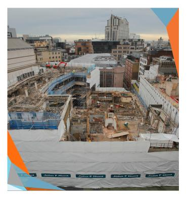
Installation and maintenance of split-level piling platform including extensive pile probing and phase 1 temporary works.
