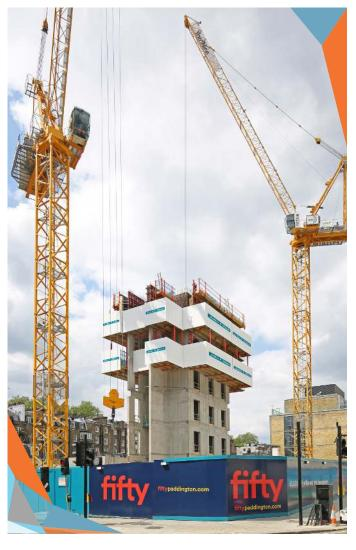
RC cores erected using Jump-Form formwork system RC concrete and metal deck used from First Floor to Roof.
