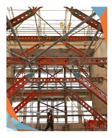
On the ground floor of the tower we removed the entire mezzanine slab and designed and installed temporary bracing in its place to make room for a deep swimming pool for residents. We demolished the existing car park ramp and filled it in to provide additional floor space for parking, with the ramp being replaced with a car lift.
