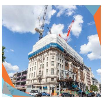
Constrained site logistics: the entire project site was serviced from a single 20m long pitlane, with limited transient material laydown areas. Due to the highly populated area and the Marble Arch elevation being a red route careful Traffic Management Plans were devised. Careful planning and collaboration were required with the party wall occupier and adjacent construction site.
